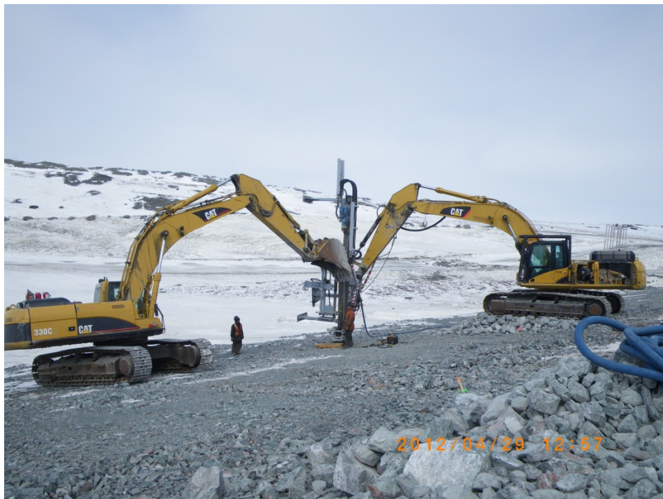
Photo 2: A sections of drill rod and outer steel casing being added to the drill stem.
