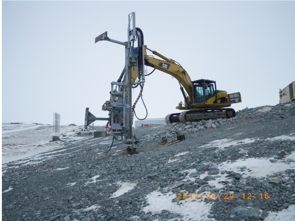
Photo 1: Drilling ND-IN-120-3 using an 330 excavator with the hoe-drill.
