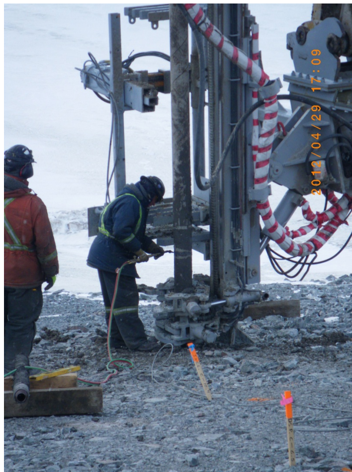
Photo 3: The outer steel casing being cut to permit removal.
